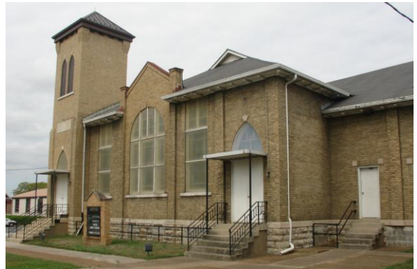
Charlotte Avenue Church of Christ, Richland Park, built in 1921, demolished by congregation in June.
